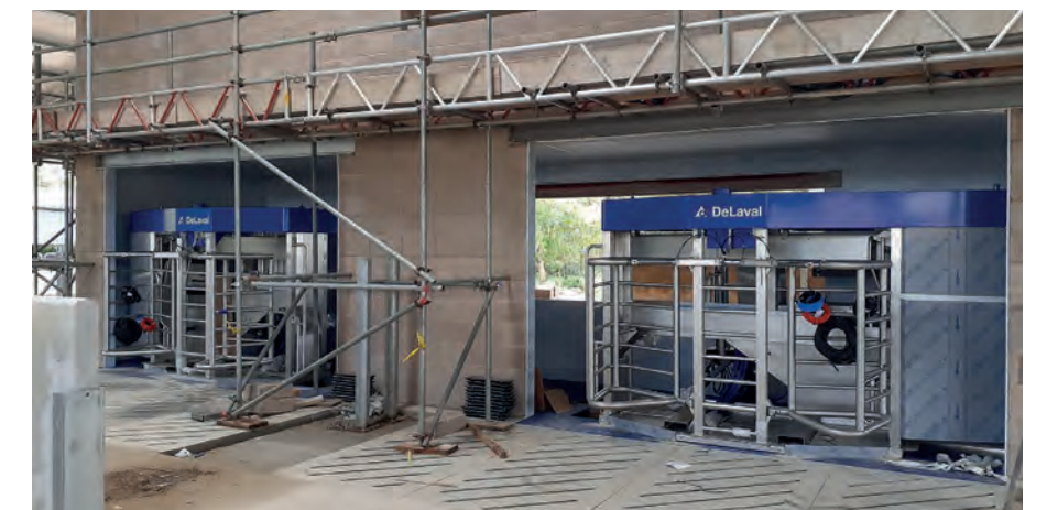
Two DeLaval VMS robotic milking units were installed in October, with a third to follow for teaching.
