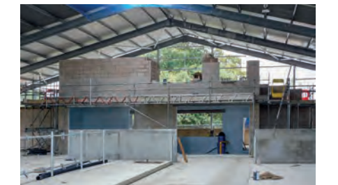
Internal structures nearing completion.
