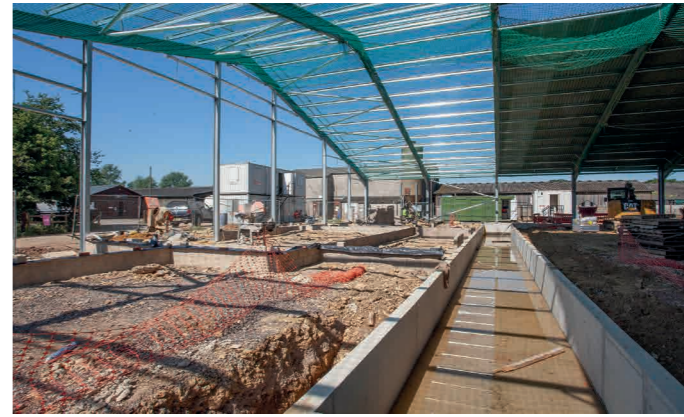
Below: Inside the building the slurry channel, as well as block walls for the VMS units and teaching spaces take shape.
