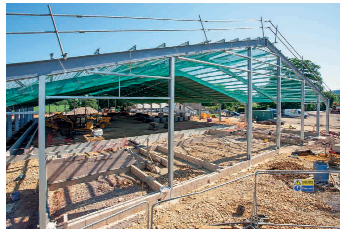
Top and above: The steel frame of the new dairy unit on the Lackham campus was well advanced in June.
