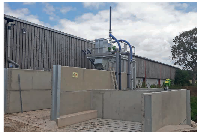
Top: David and Tom Johnson are delighted with their new separator, which has been in use since April 2019. Above: Two views of the installation under construction.
