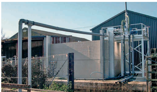
Top: Arthur Rolf, moving towards self-sufficiency in fertilizer. Middle: FAN 1.2-780 Above: The completed installation
