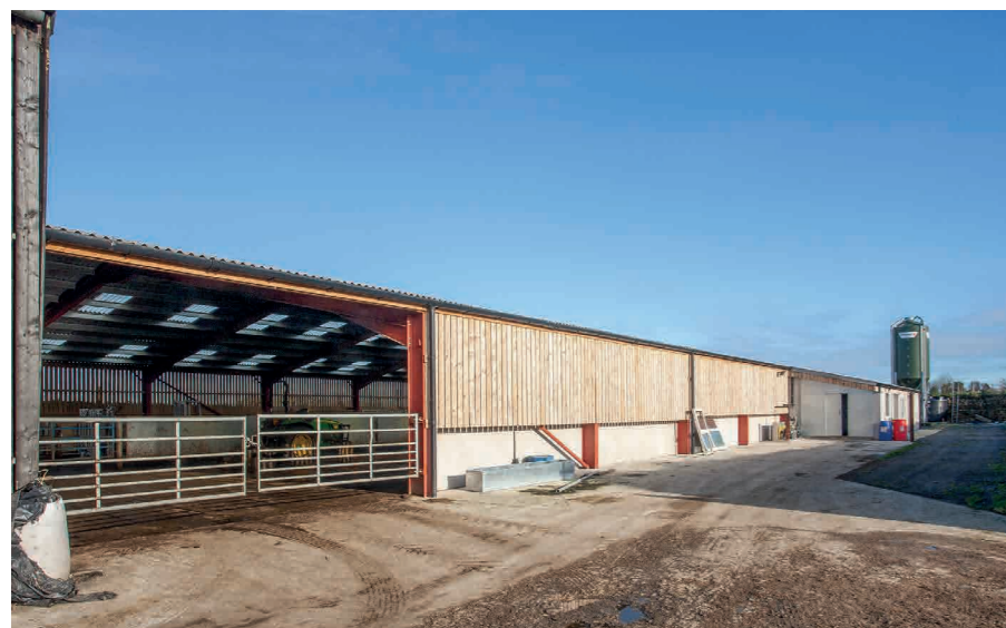
Top: Tom and Jonathan Osborne in their new parlour. Above: The large new shed housing the parlour.
