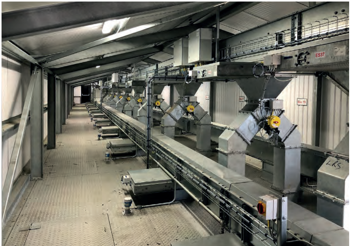
Above: Conveyors over the top of the silos in Crisp Maltings' new plant. Below: The process area.
