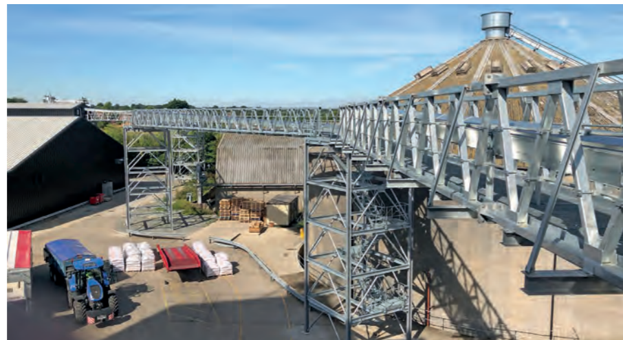
The plant's steelwork towers and gantries were fabricated by T H WHITE Projects.
