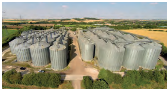
The Linton APC was the first to be built by T H WHITE for Camgrain.
