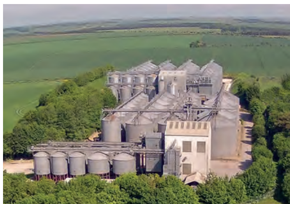
Trinity Grain's 100,000 tonne grain store at Shrewton – the original 30,000 tonne facility in the foreground with the extension beyond.
