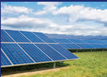
Solar park maintenance and surveillance
